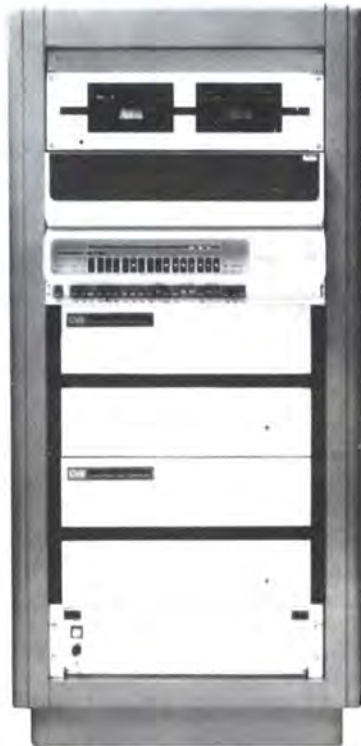
Figure 4: All EPIC components, except the compact keyboard, can be housed in a single 19" rack.
